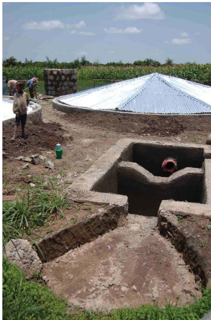
Water storage under construction
