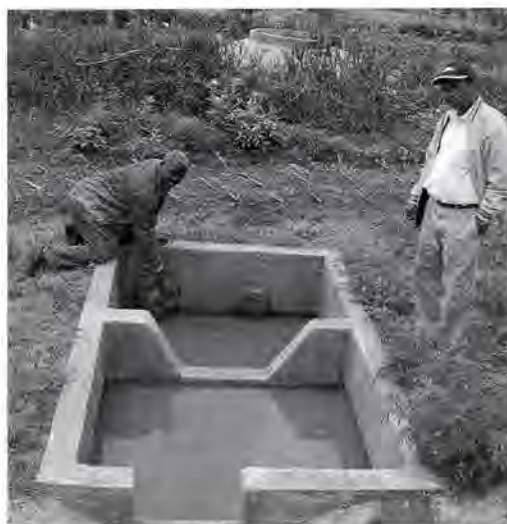
Fig 4. Silt trap with two siltation chambers.
